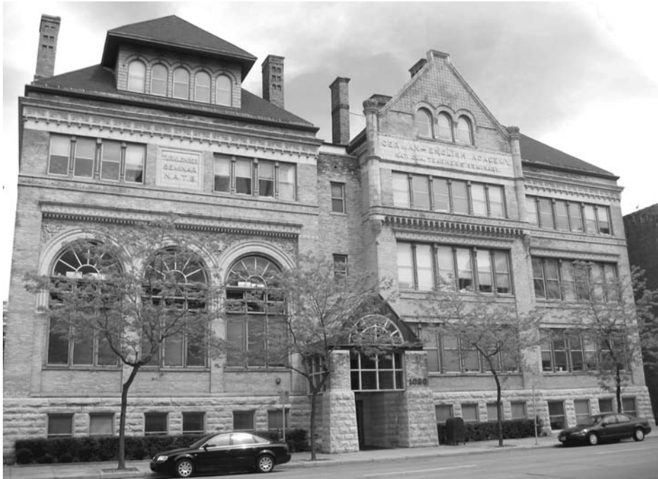
The German-English Academy building in Milwaukee as it appears today.
